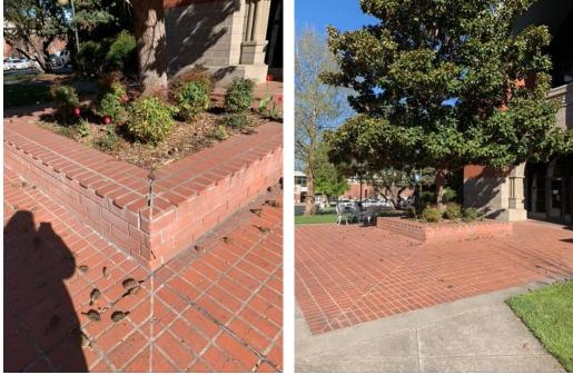
Note: deterioration of the planter and sidewalk leads to accessibility issues
